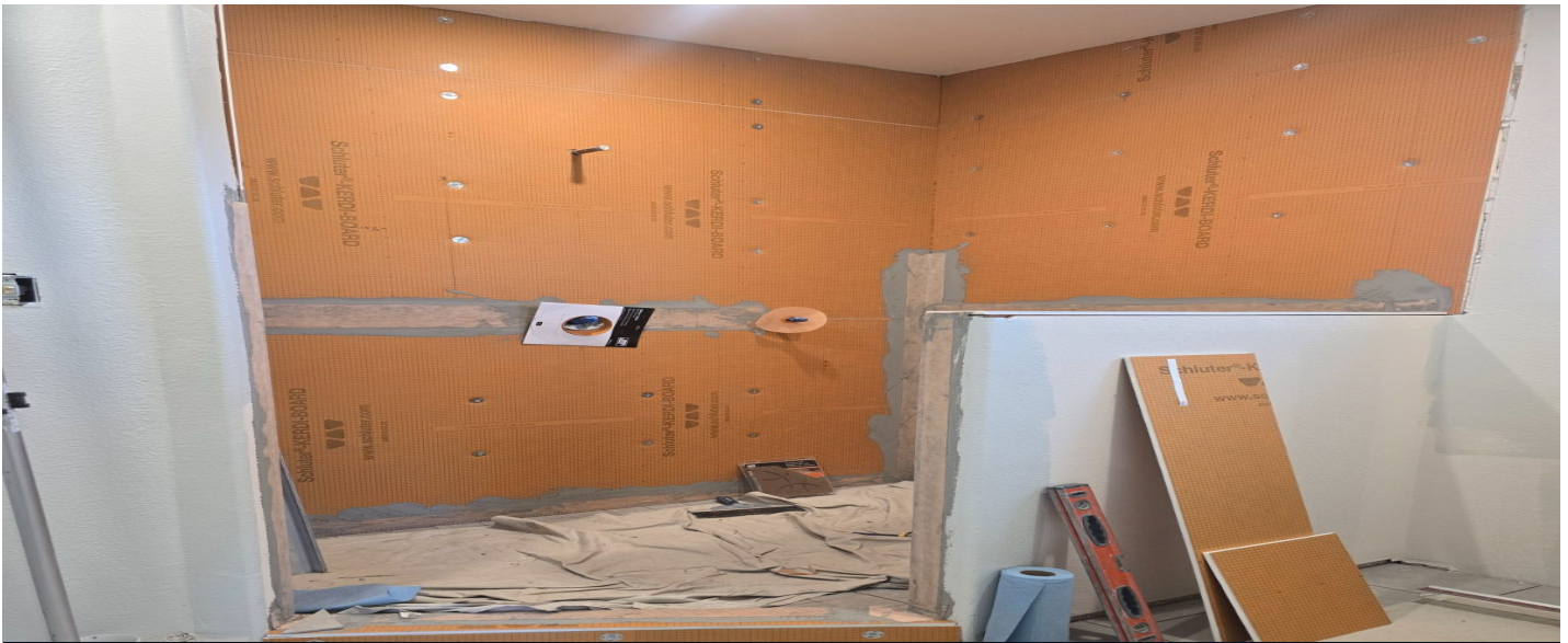
PHOTO 4 — WATERPROOFING COMPLETE
