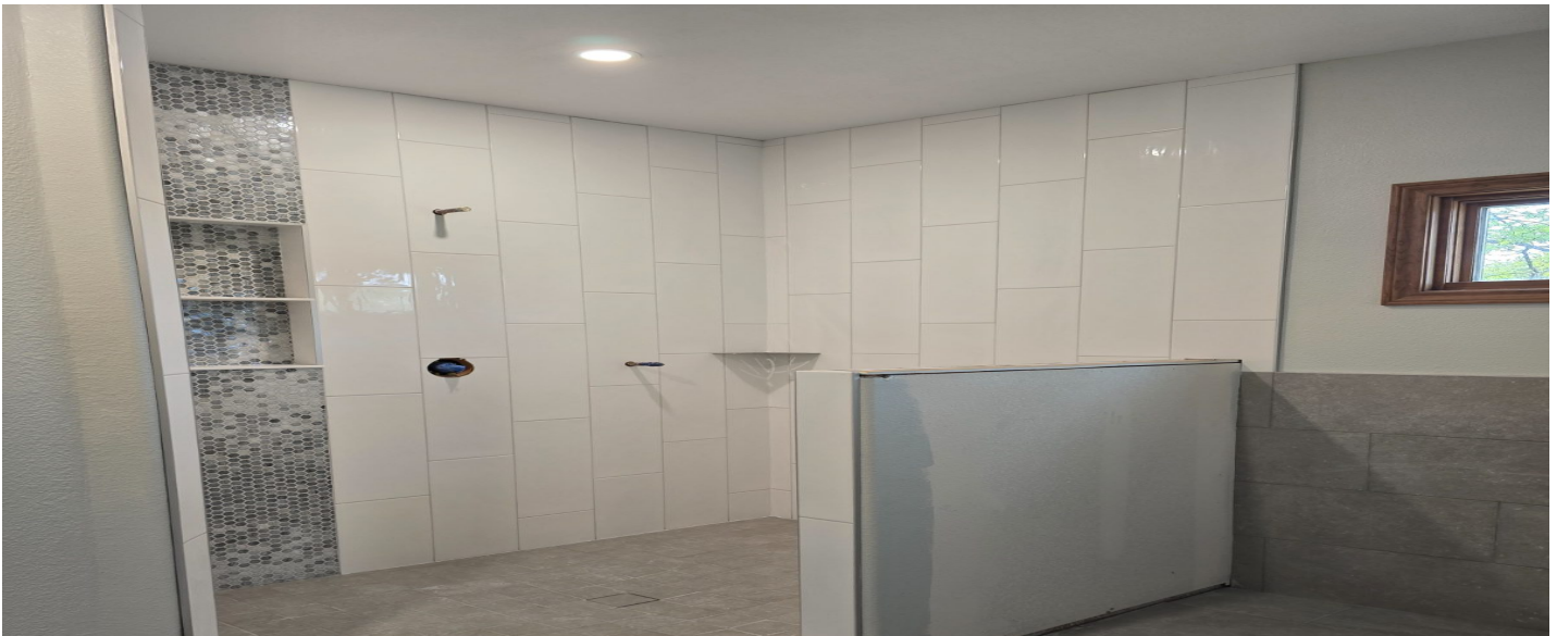
PHOTO 13 — COMPLETE TILE INSTALLATION
