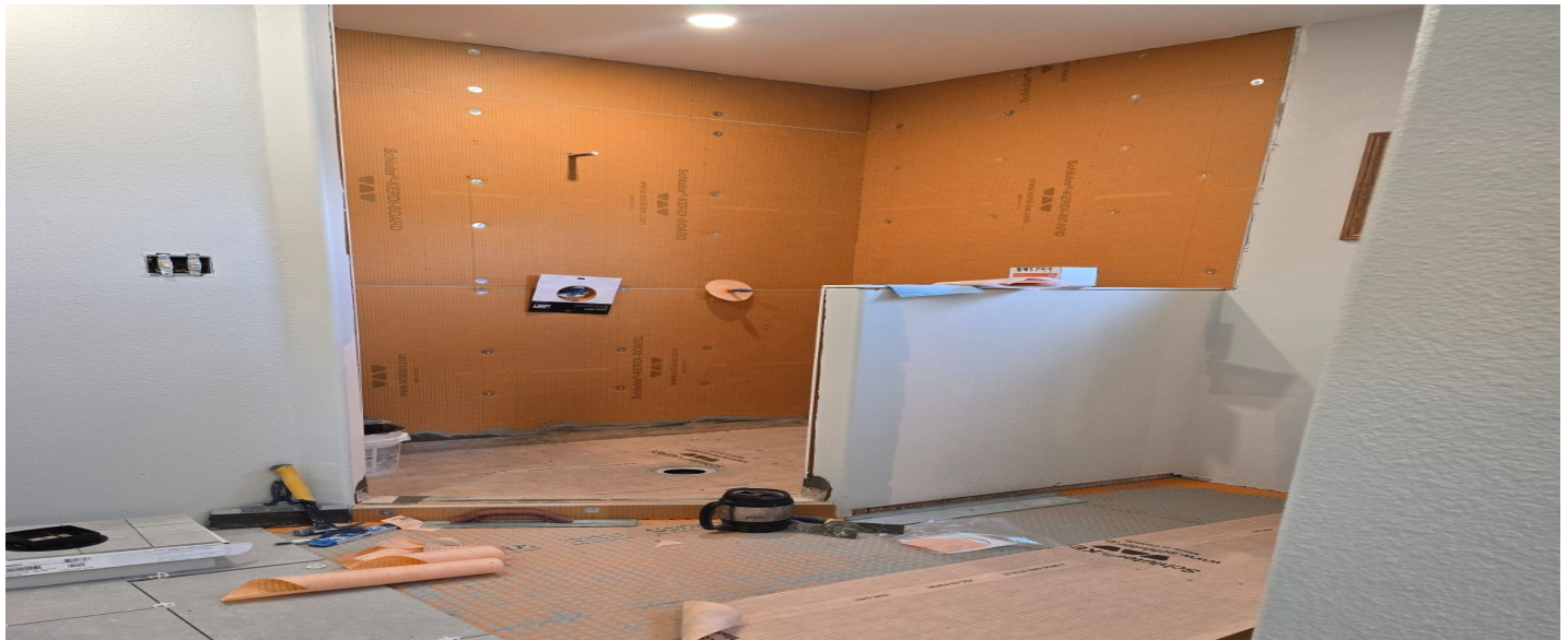
PHOTO 1 — KERDI BOARD INSTALLED
