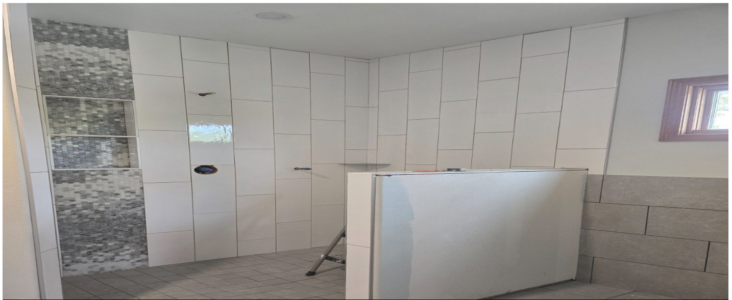
PHOTO 10 — TILE INSTALLATION COMPLETE
