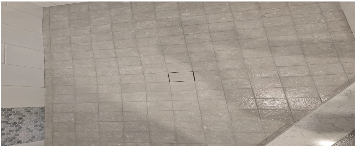
PHOTO 11 — TILE SHOWER BASE, TILE DRAIN COVER
