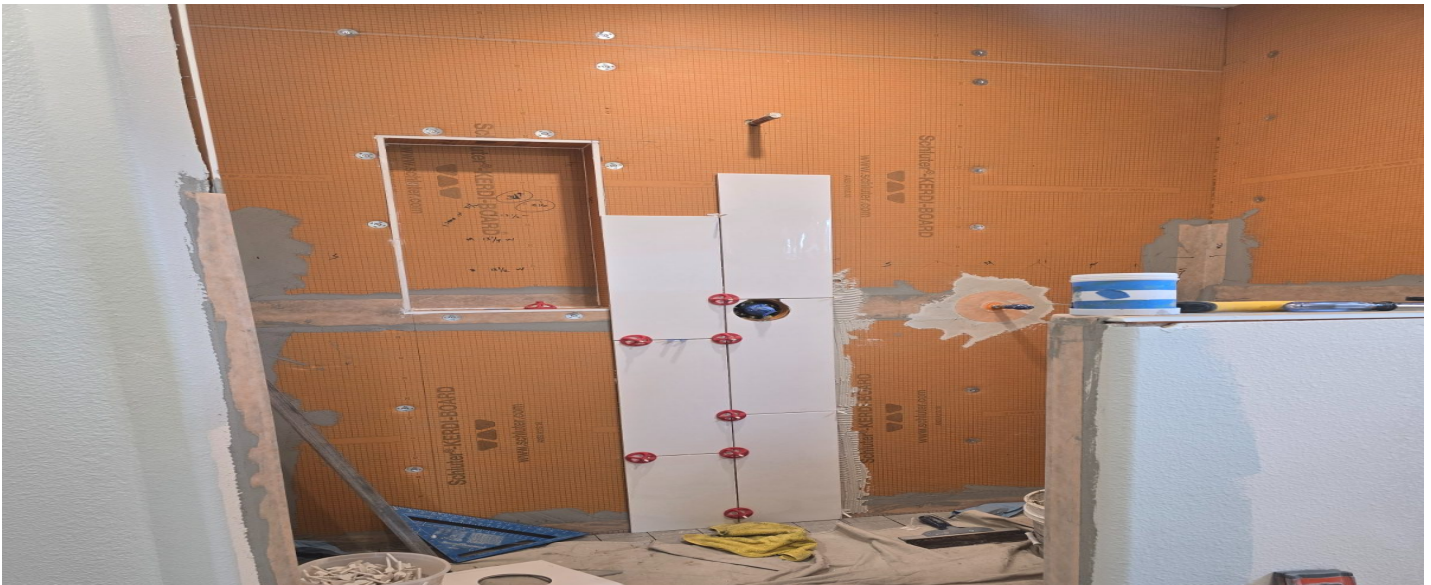
PHOTO 5 — BEGINNING TILE INSTALLATION
